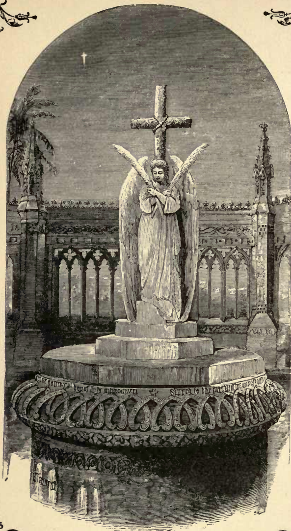
INTERIOR OF WELL AT CAWNPORE.
